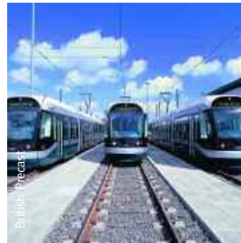
Stanton twin block concrete sleepers
