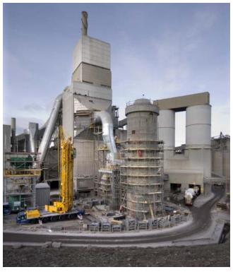
Construction of specialist equipment such as this gas scrubber has radically reduced sulphur dioxide emissions
